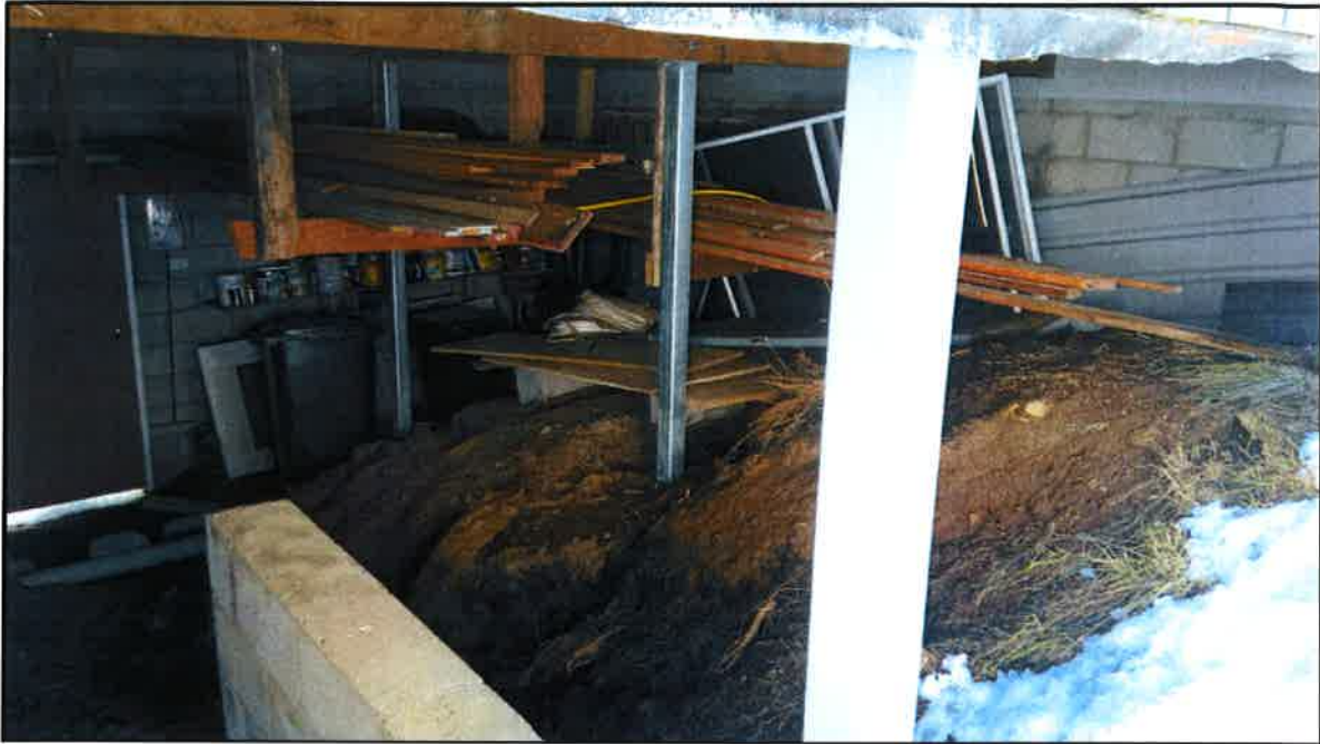
Figure 3: Space to be excavated for bedroom (Source: Department site inspection photo)
